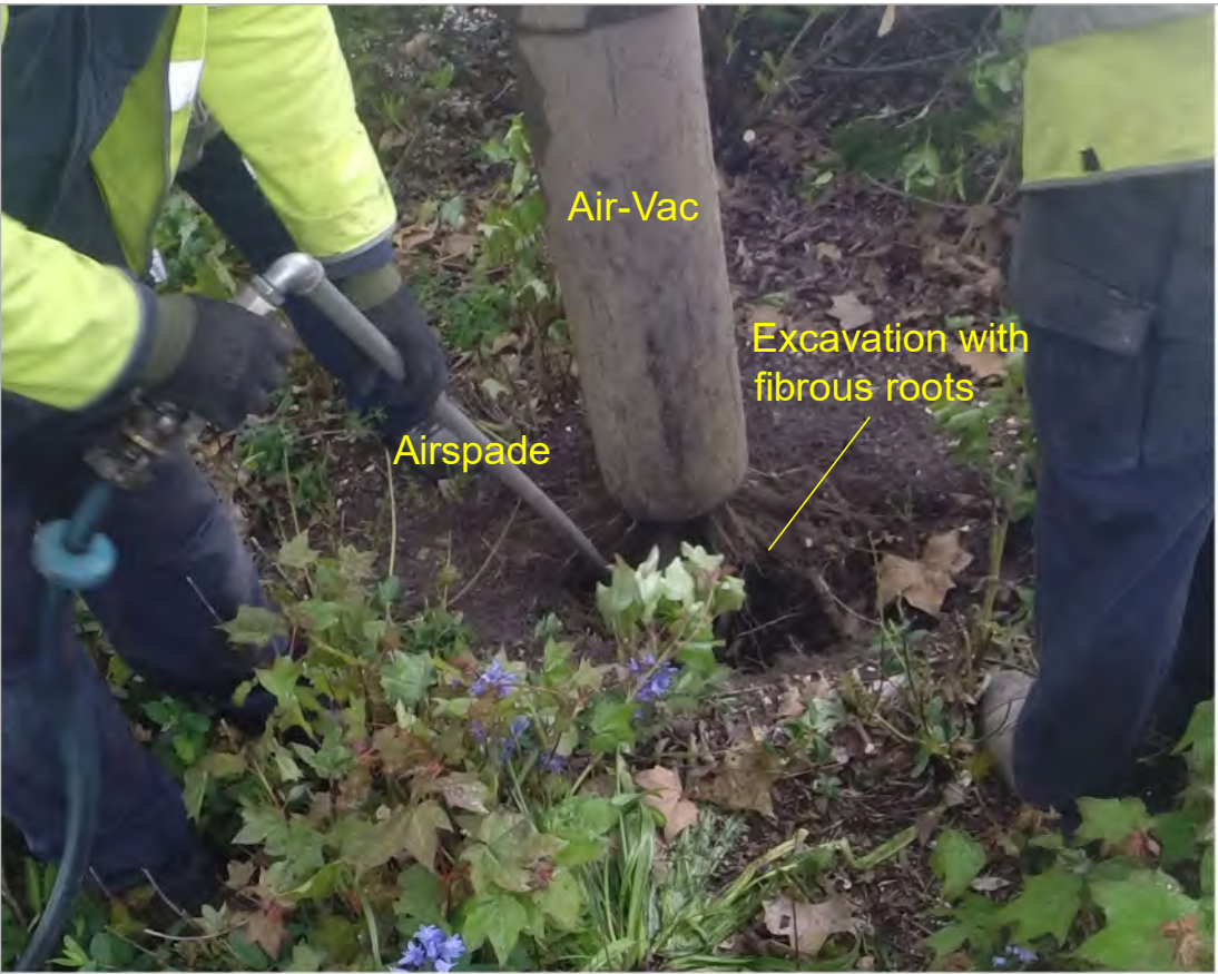
Figure 1 - Air spade application with air-vac truck
