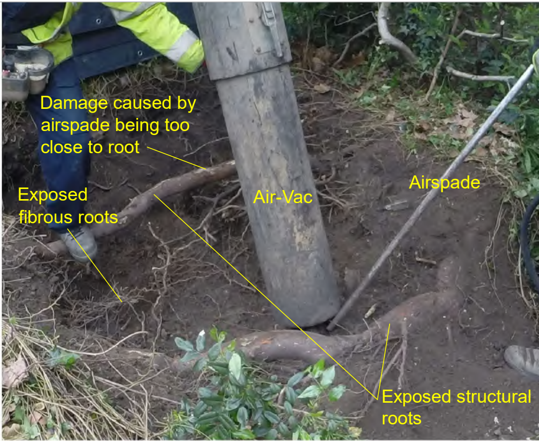
Figure 2 - Air spade exposing large structural roots
