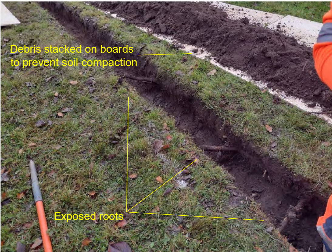
Figure 3 - Airspade with no air-vac truck, boards used to store soils
